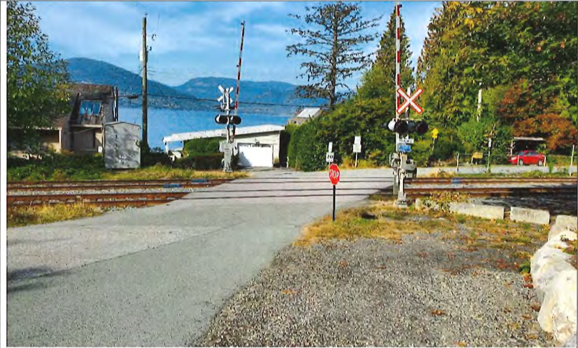
Brunswick Beach Avenue Railway Crossing, Westbound Approach (Stop Signs to be Removed and Narrow Lane Widths)
