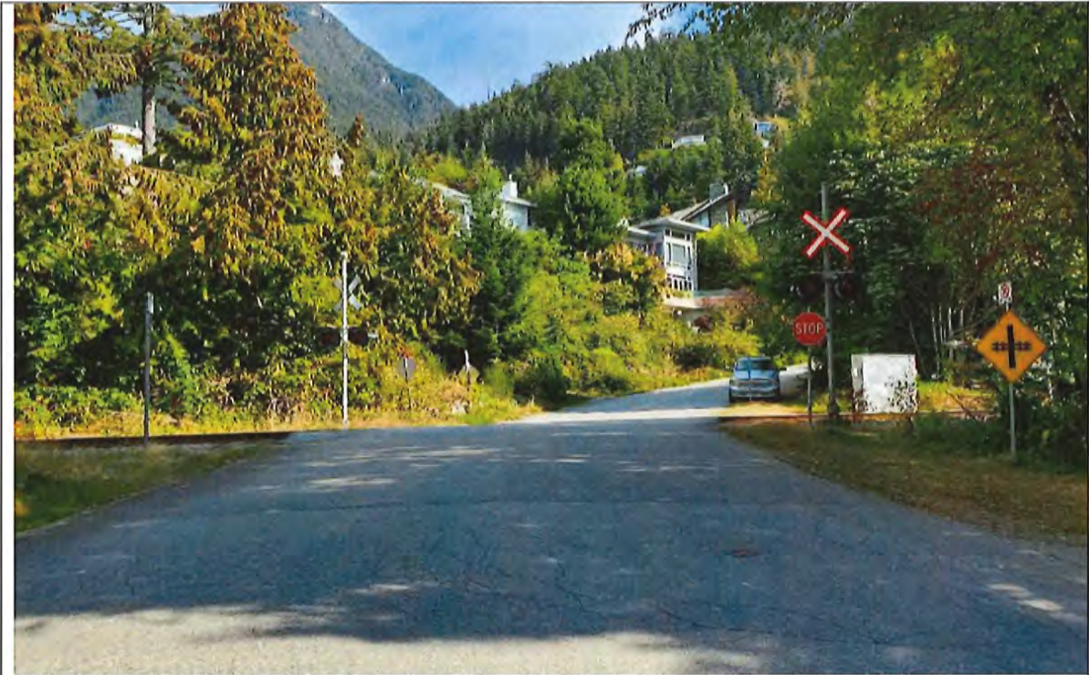
Tidewater Way, Eastbound Approach (Stop Signs to be Removed)
