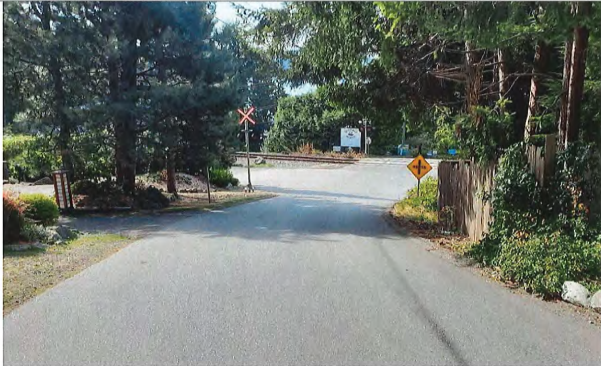
Lions Bay Avenue, Westbound Approach (At Decision Sight Distance for Proposed 20 km/hr Posted Speed)
